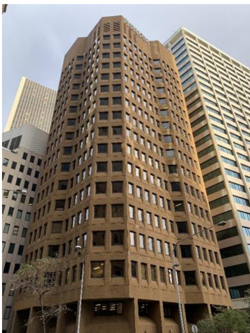
Figure 18 – Building at 3 Spring Street, viewed facing west at intersection of Spring & Gresham Streets.
